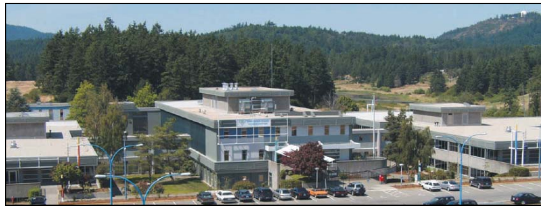
Figure 1: Vancouver Island Technology Park
